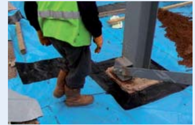
Make sure the root barrier membrane is sealed properly around pillars and other structures.
