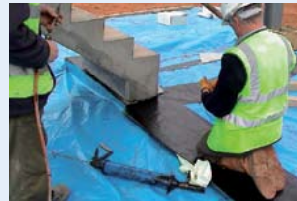
Make sure the root barrier membrane is sealed properly around pillars and other structures.
