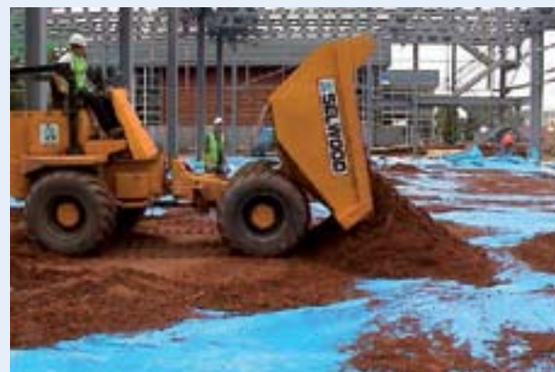
Stage 3: Apply another layer of sand over the surface of the root barrier membrane.
