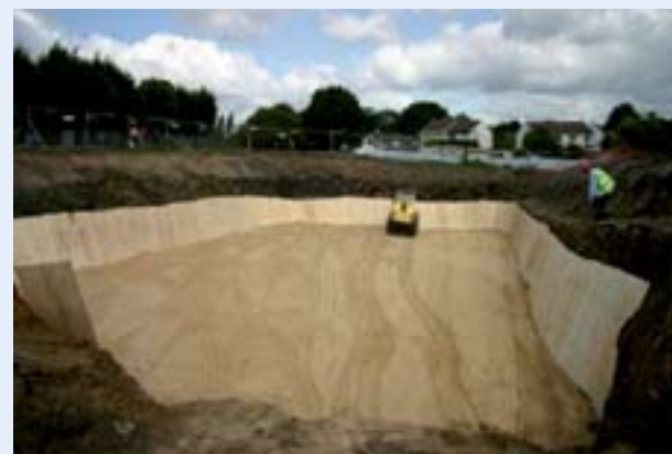
Stage 2: Protect the integrity of the root barrier membrane with a layer of sand and provide shutter ply supports for the edge of the cell.
