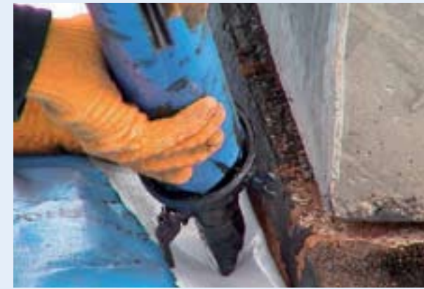
Make sure the root barrier membrane is sealed properly around pillars and other structures.
