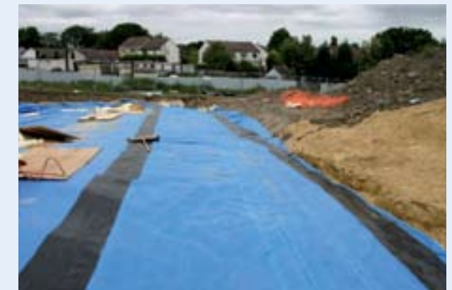
Stage 8: Protect the surface of the cell with sand and bury deep enough to prevent disruption in the future.
