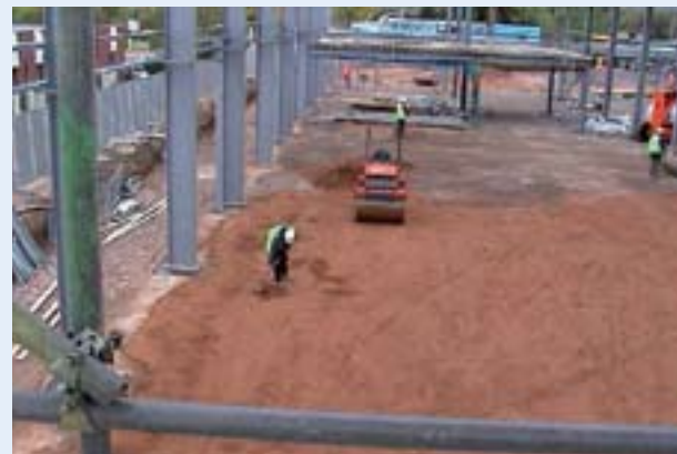
Stage 1: Protect the integrity of the root barrier membrane and prevent damage from 'heave' with a layer of sand.
